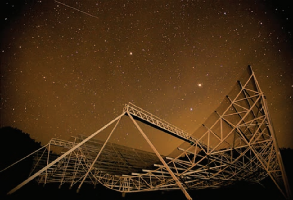
Figure 1 – Walkways suspended above each reflector in the CHIME telescope carry the dual-polarization feeds and low-noise amplifiers.
