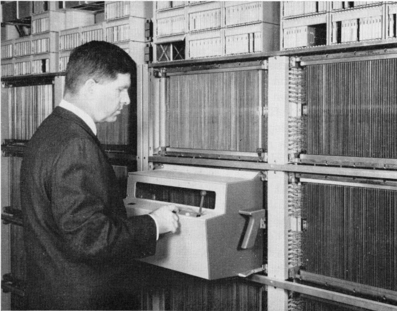
Fig. 29 — Card loader in use on program store.
