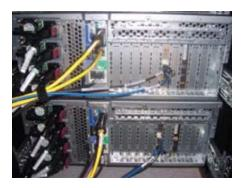
**Figure 2.** Configuration of the server wiring when two 10G connections replace eight 1GbE connections.
