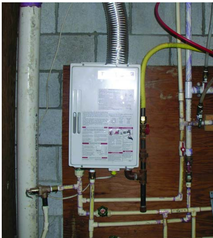
Figure 1. Takagi Tk Jr 144K BTUH Hot Water Heater
